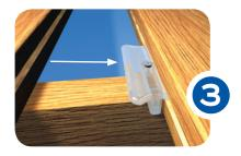
Step 3: Slide next deck board into place. Now tighten the screw.
